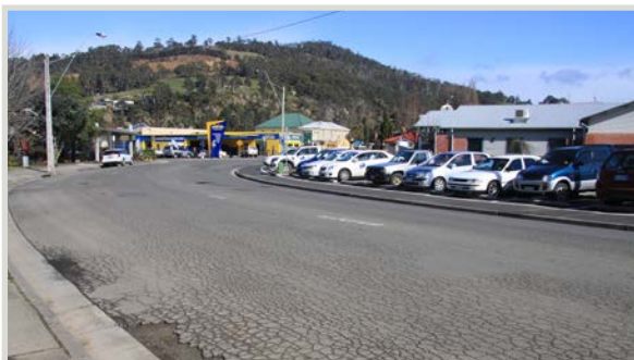
Sale Street in Huonville before reconstruction
