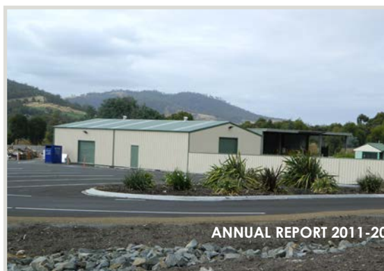
Improvements to Southbridge Waste Transfer Station and the new Reuse Shop
