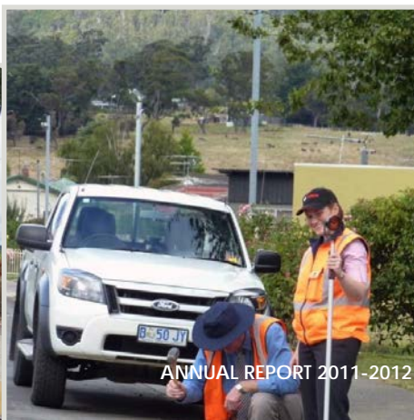
Surveying roads for reconstruction
