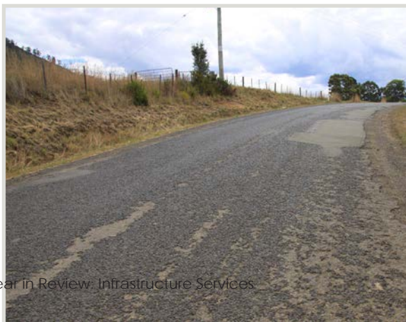
Lonnavale Road before reconstruction
