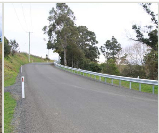
Lonnavale road after reconstruction
