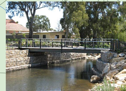
Example channel wideing and erosion control
