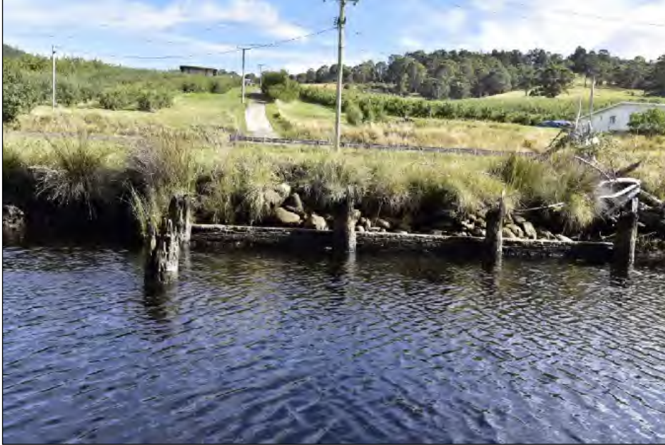
Plate 28 Powerlines and previous retaining works within the narrow portion of this section
