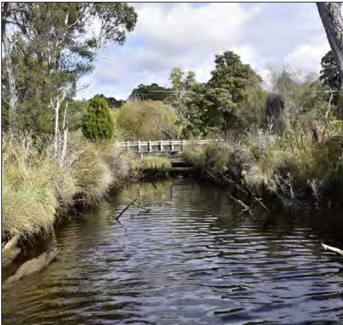
Plate 35 A bridge is required over Clarks Rivulet
