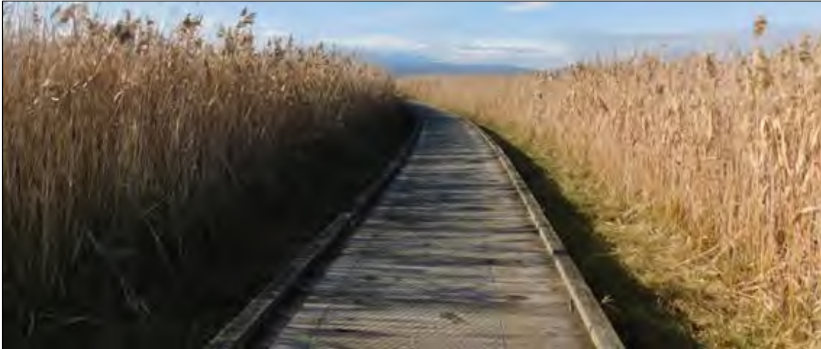
Plate 50 Example board walk with side rail and slip prevention wire (from Tamar Wetlands)
