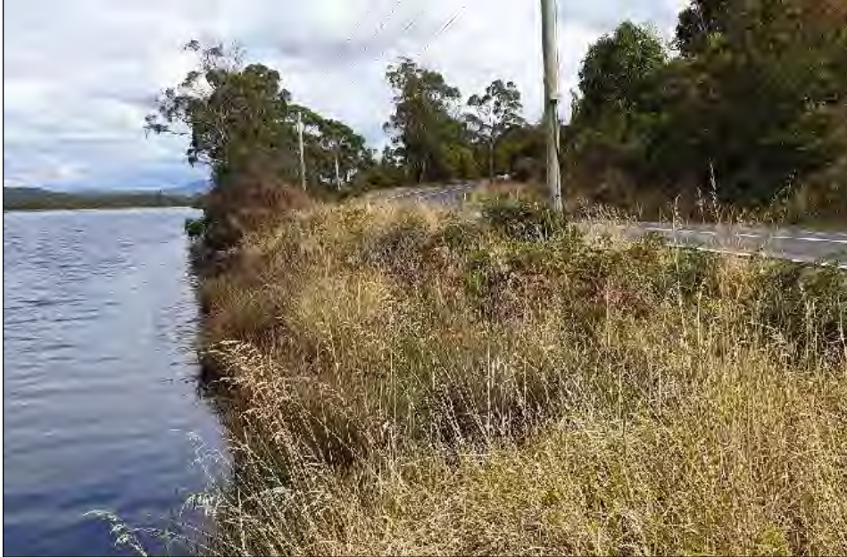
Plate 36 Proximity to the road limits the area available for construction
