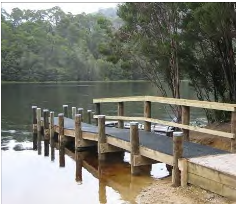
Plate 51 Example jetty with FRP surface and pine superstructure (Source: Grating Tasmania)
