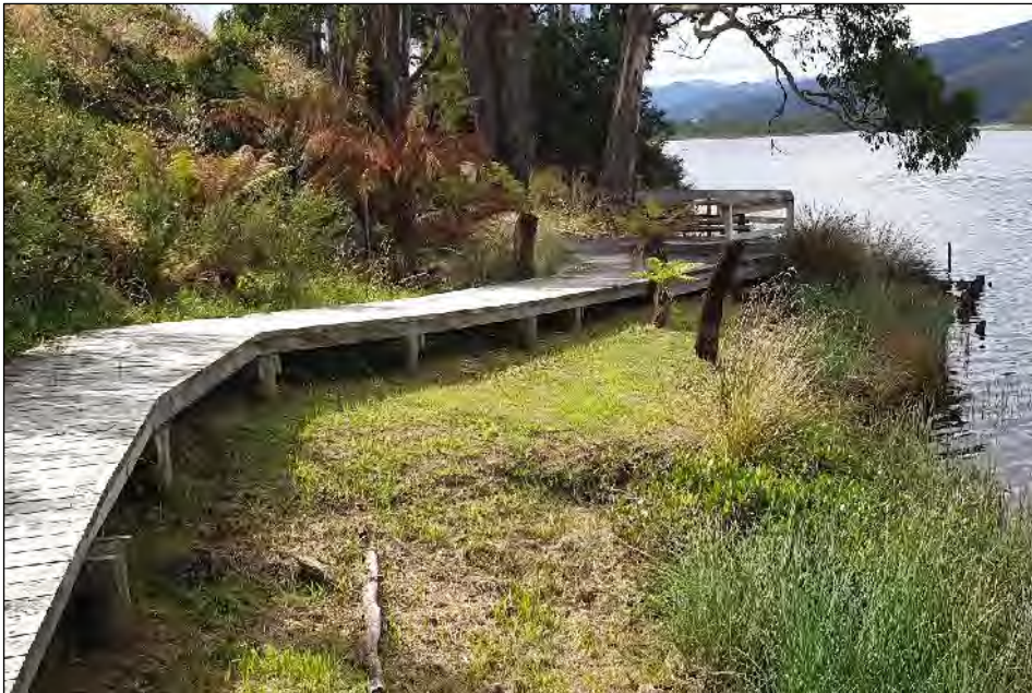
Plate 45 The current path is constructed of treated pine
